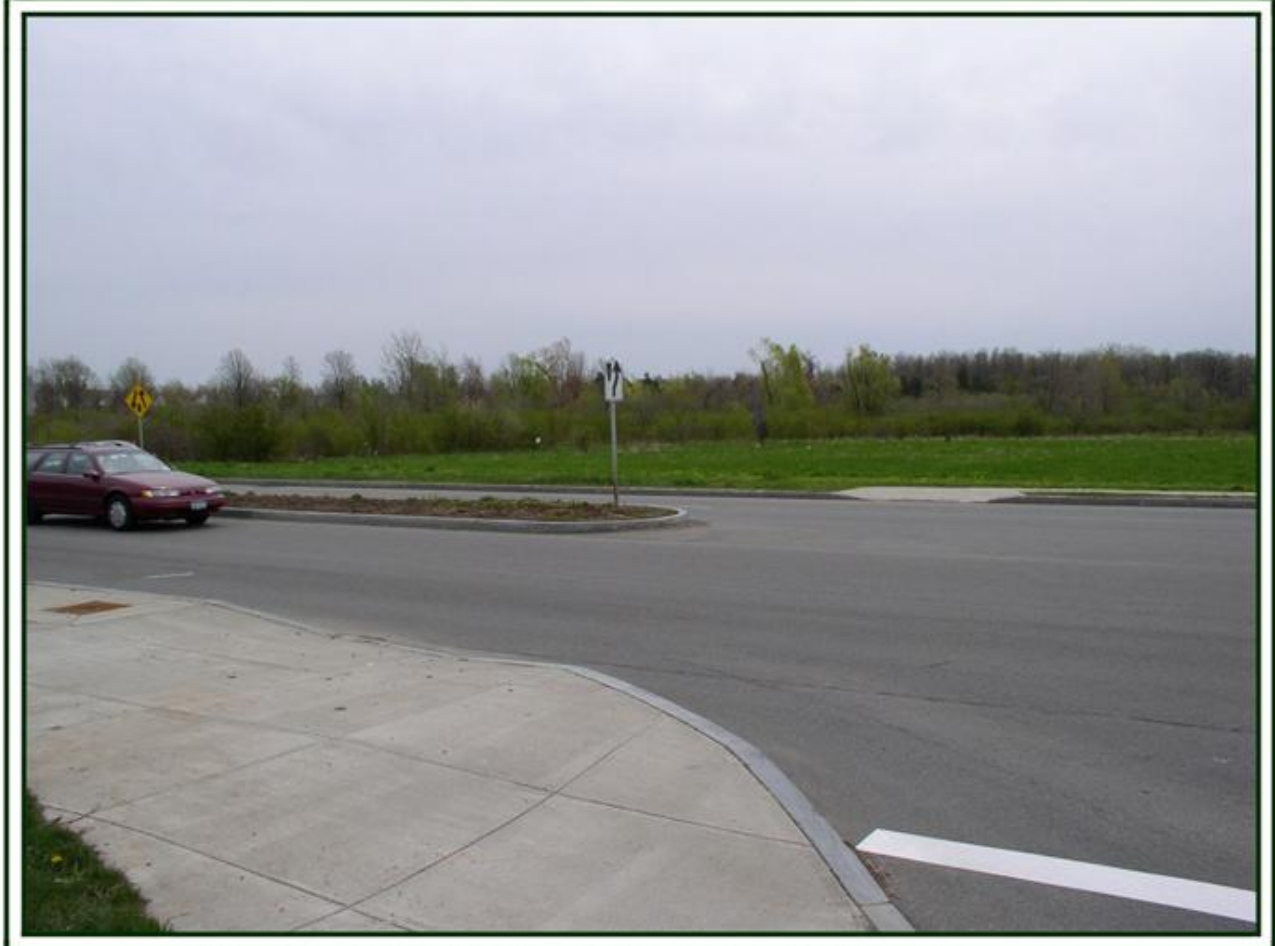
VIEW No. 7: ELMWOOD AVENUE TRAIL CROSSING AT GOODMAN STREET - EXISTING CONDITIONS PREPARED BY: McCORD LANDSCAPE ARCHITECTURE
