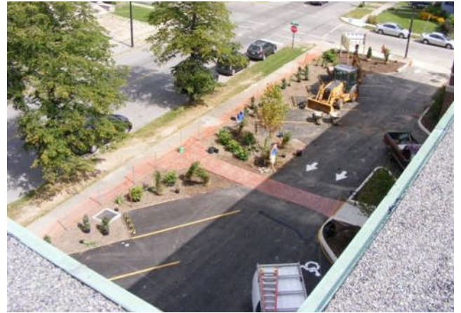
Off-street parking lots can be designed with pedestrians and aesthetics in mind.
