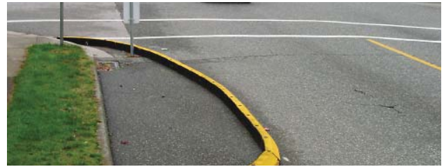
Temporary Curb Extension
