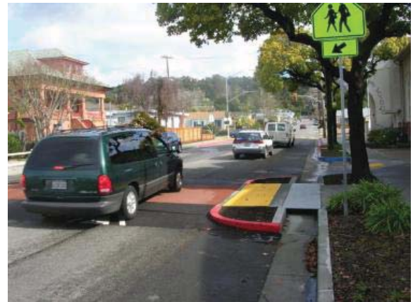
This raised crosswalk incorporates curb extensions that facilitate drainage. Source: East Bay Bicycle Coalition
