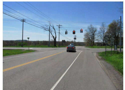
NYS Route 15A Intersection (Looking West)
