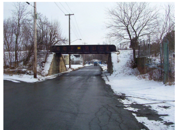
Gates Ave. Railroad Crossing
