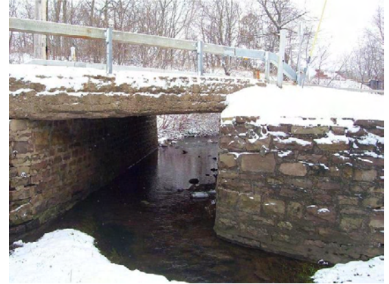
Box Culvert along Veterans Drive
