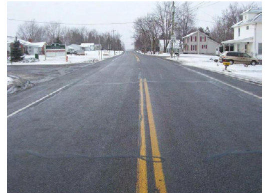
Rte 31 at the Holley Industrial Park
