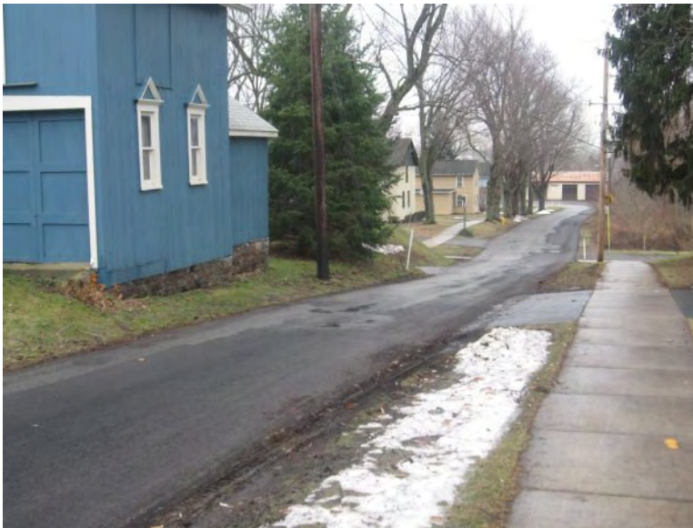
Figure 16. North Street looking south toward former railroad crossing. Note proximity of blue building on east side of road (photo left) and road narrowing to single lane north of alignment.
