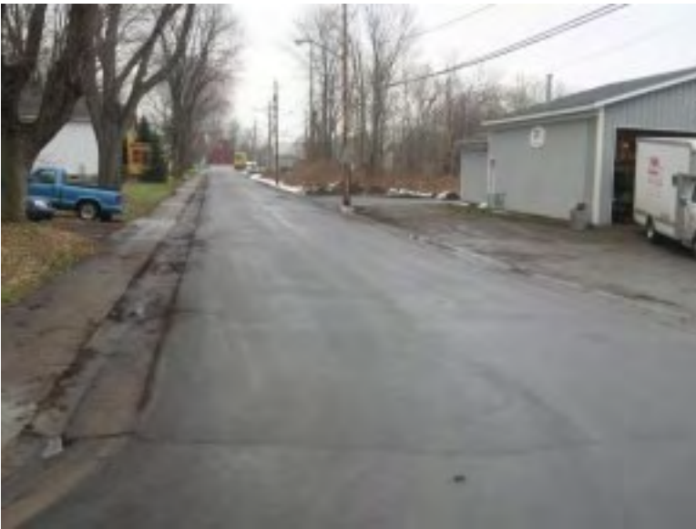
Figure 14. Howard Avenue looking east toward the Bean Mill (red building in center background)
