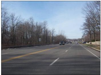
Where the sidewalks end along Route 5, shoulders become wider (eight to ten feet in width) with larger property setbacks for roadway drainage. Many properties have multiple access points, large amounts of pavement, and vary in setback. The pavement exhibits some longitudinal cracking with sealing and edge cracking along the shoulder.
