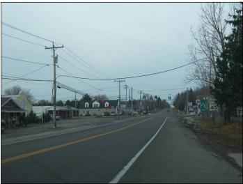
Route 33 begins as a two lane roadway near the Town line with wide shoulders (6-10 feet wide) and no pedestrian facilities. Pavement condition is generally good with cracking observed near the edges.
