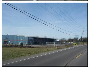
Bordering and within the City, large commercial and industrial uses line Route 33. Lots are much larger in size, with parking areas of equal size. Setbacks are much greater and buffering against the roadway consists of grass. The structures consist of pole barn-type and concrete block construction.
