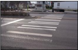
These two images from Batavia show instances where pedestrian island refuges would be beneficial to protect pedestrians from traffic. The bottom image also shows where regular maintenance of sidewalks is important as the markings will where down over time.
