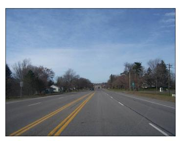
East of the City of Batavia, Route 5 begins as a four lane roadway and is lined with a mixture of residential and agricultural uses. Shoulders are wide (6-10 feet) and are utilized by pedestrians or bicyclists. Pavement is generally in good condition with slight longitudinal cracking observed; drainage is provided by roadside ditches.
