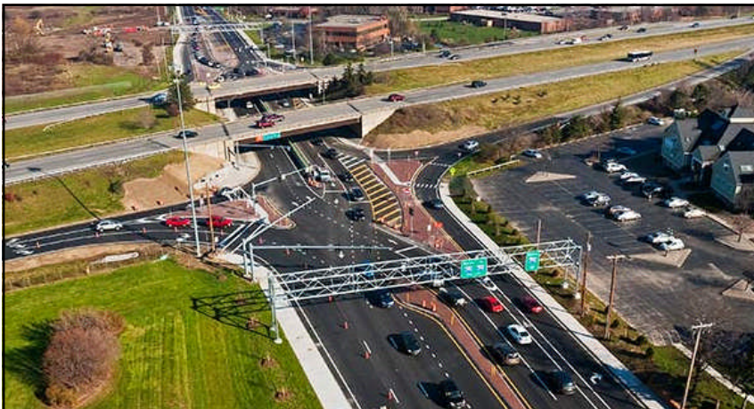
An aerial view of the Diverging Diamond Interchange at the junction of I-590 and Winton Road in the Town of Brighton. Opened in October 2012, this is the first Diverging Diamond Interchange in New York State.
