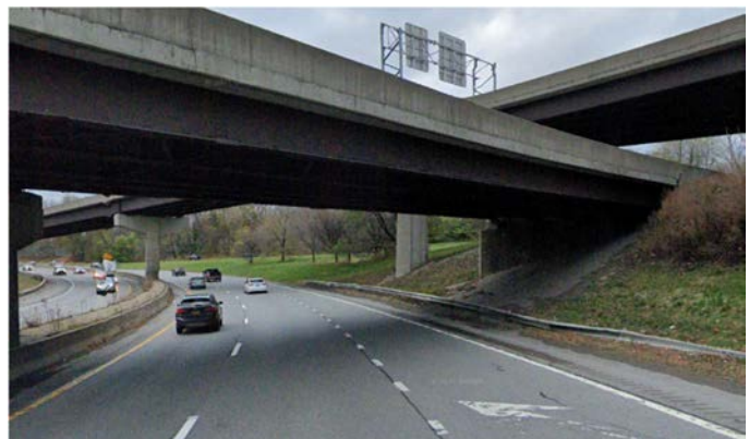
Exhibit 2.1.3.A-1 Brick Paved Slope and Bridge Abutment / Pier Adjacent to Ramp WS, Source: Google Street View
