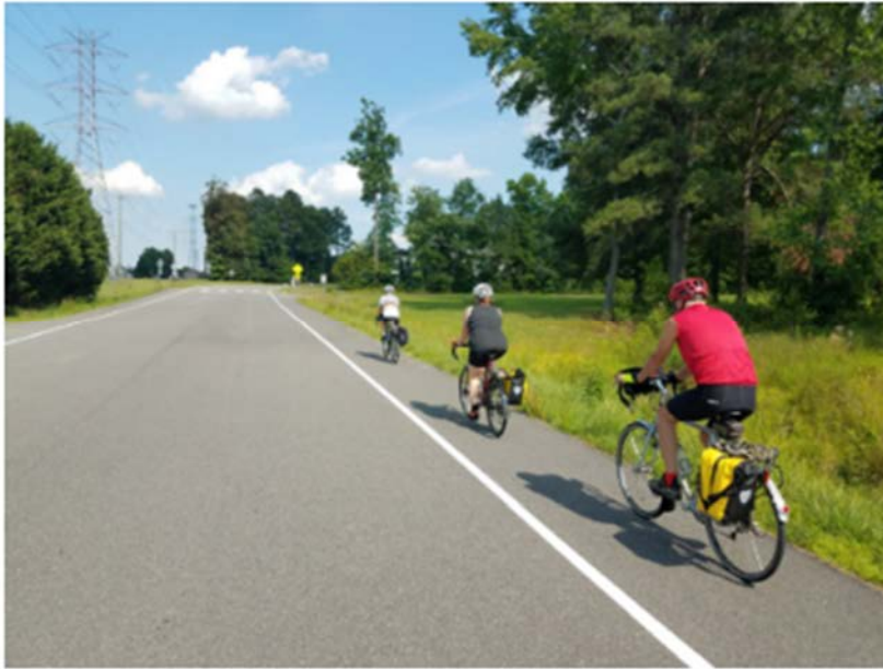
Exhibit 9 – AASHTO GDBF - Figure 12-2: Example of a Paved Shoulder
