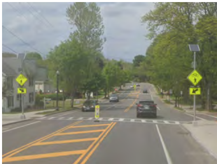
Rectangular Rapid Flashing Beacon (RRFP) and High Visibility Pedestrian and Bike Crosswalk
