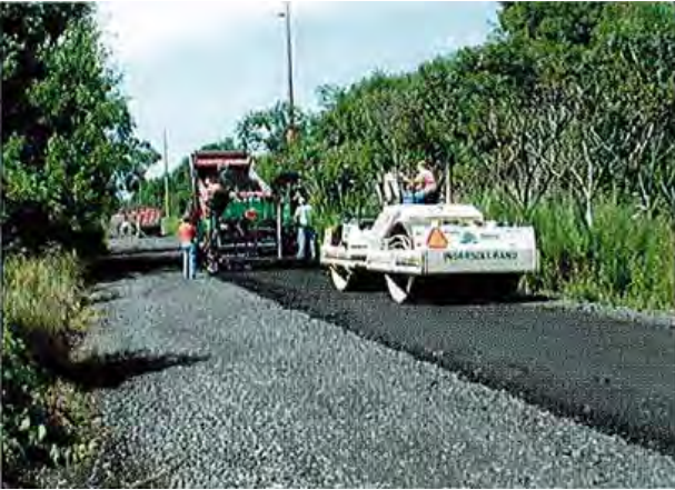
Laying & Compacting the Cinder Trail Base
