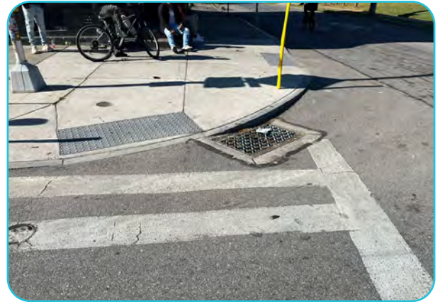
Intersection of Wilkins and Joseph: drainage inlet near base of curb ramp; detectable warning surface.
