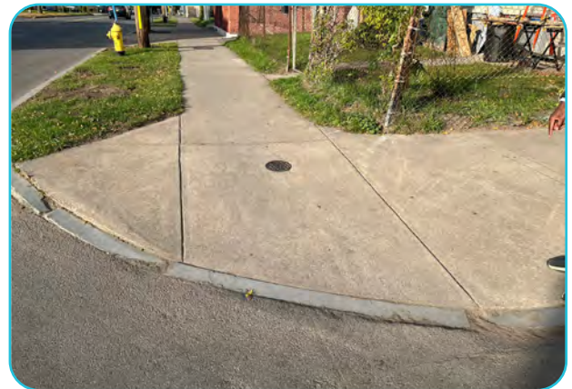
Intersection of Laser and Joseph: Curb ramp without detectable warning strip.
