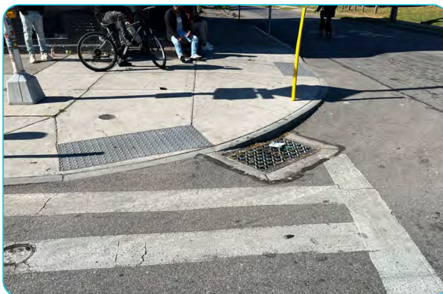
Existing conditions: Newly installed curb ramp on southwest corner.
