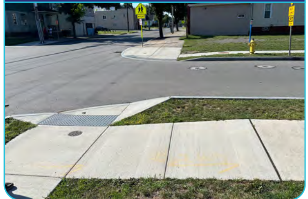
New curb ramps with detectable warning surfaces at Weaver and Joseph Ave.
