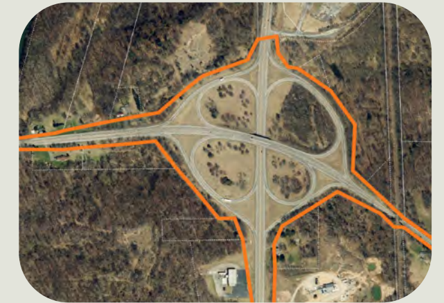
Photo: Route 96 over Route 14 Interchange Project Area
