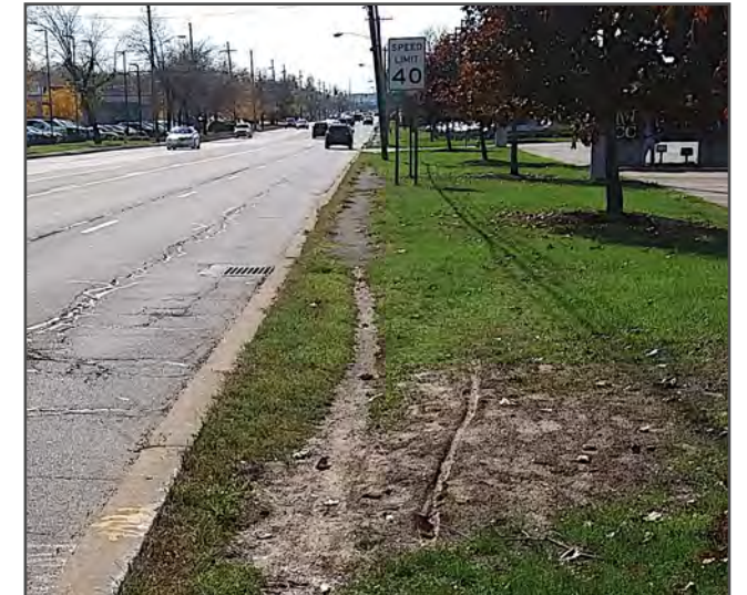
Desire paths are observed along many high-speed roadways, indicating that there is pedestrian demand despite a lack of safe facilities
