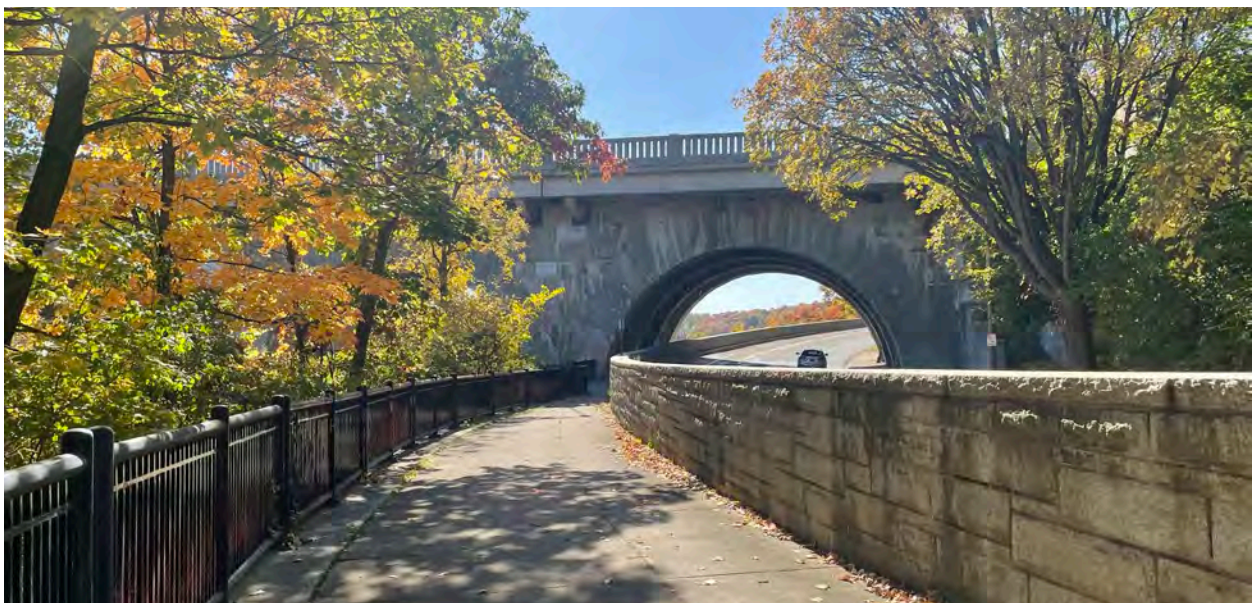
Bridge View Road Diet Existing Conditions looking South
