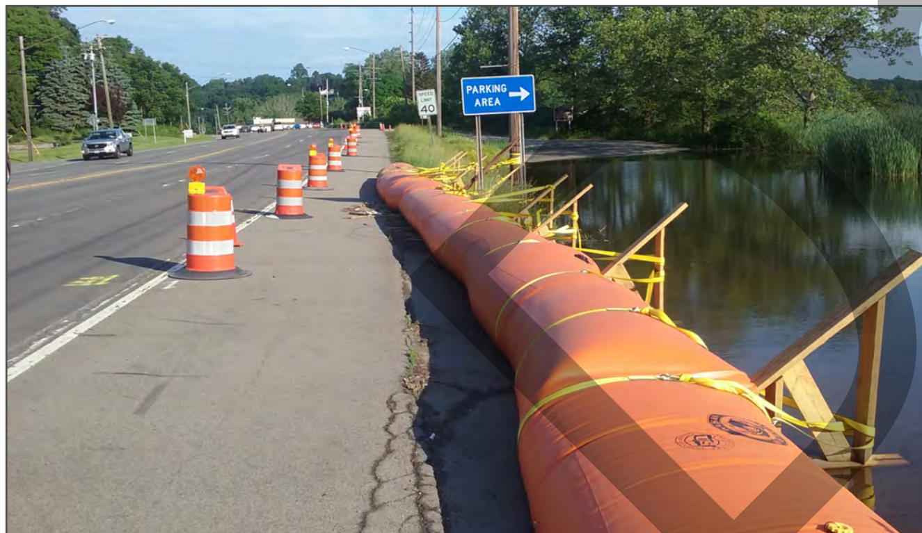
In 2017, a temporary dam was erected along NYS Route 404 (Empire Boulevard) at the southern end of Irondequoit Bay to protect the road from high water levels
