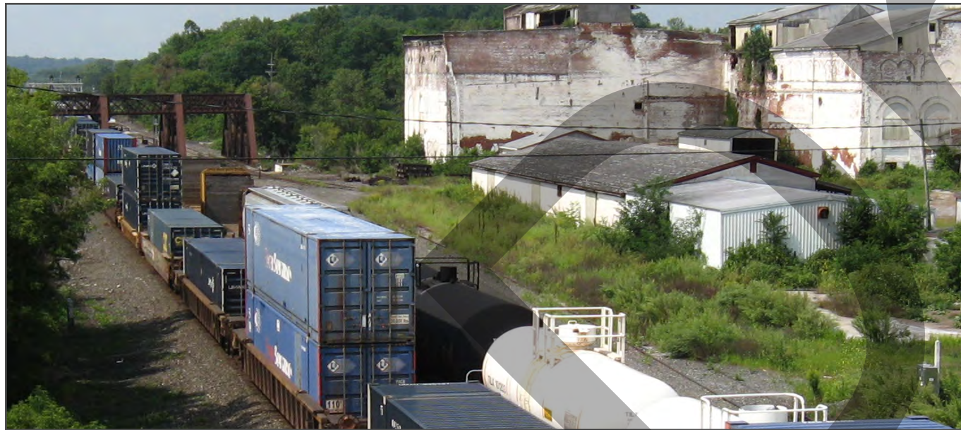
CSX Mainline Class I Railroad in Lyons
